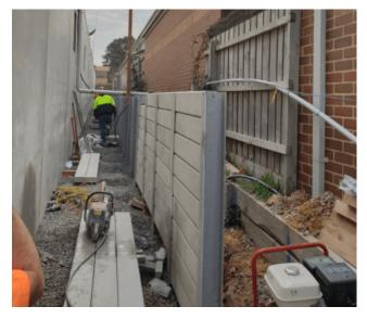
Panel and post retaining wall systems have long been regarded as one of the most straightforward to construct. To build the wall, the concrete posts are first inserted into the ground to form the frame, and then the blocks are slid into place.
