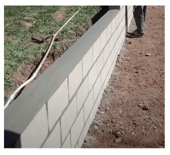
blocks. A block wall will usually have less load-bearing weight and should not be used to hold back large amounts of weight and earth.
