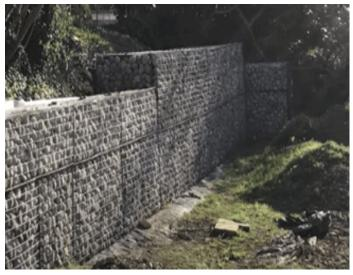
and long-lasting, and they prevent soil erosion and flooding, making them a smart long-term investment. A gabion wall can be used as a residential retaining wall in your backyard in a smaller size.
